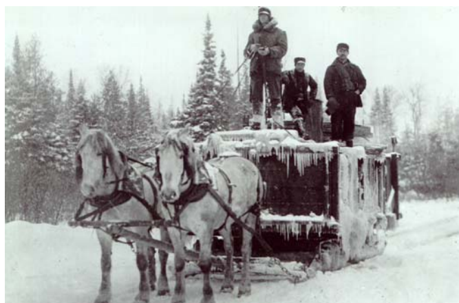
Ice road sprinkler sleigh with Andy McGinnis. Sleighs hauled and sprinkled tanks of water over the roads to ease the hauling of log loads. One team of 20 men would pack the snow before water was sprinkled on the road.
