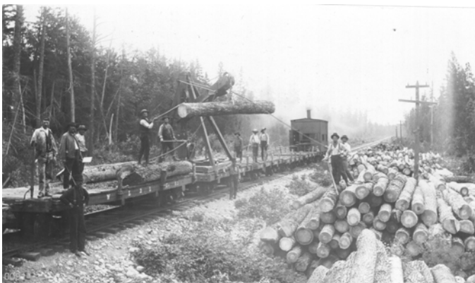
Loading logs about 7 miles east at Farnum. Loading logs on the Soo Line with the old Austrian Loader.
